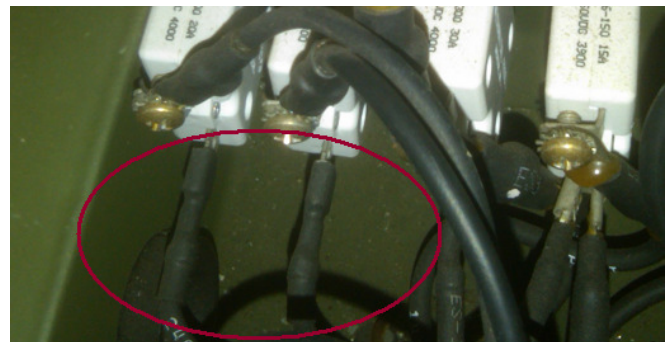
Image 2b. - "Faston" Connectors at Circuit Breakers #22 & #23
